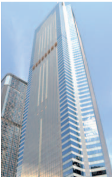
Central Plaza 18 Harbour Road
